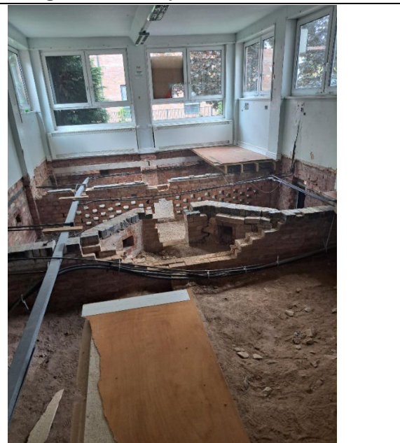
Image 6: Hinckley DH Interior post asbestos removal
