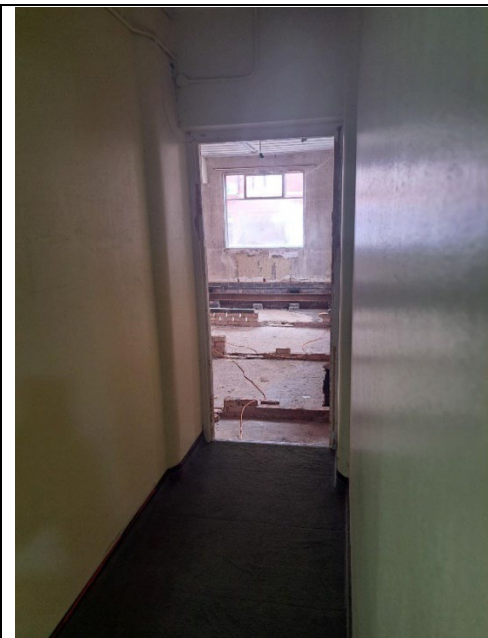
Image 7: Hinckley DH Interior post asbestos removal
