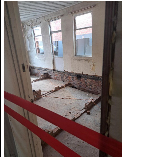
Image 5: Hinckley DH Interior post asbestos removal
