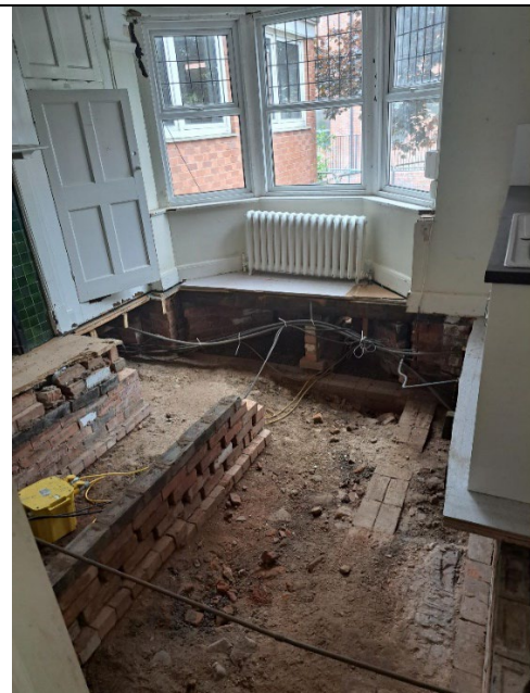
Image 8: Hinckley DH Interior post asbestos removal
