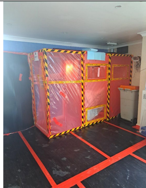
Image 10: Hinckley DH Interior post asbestos removal
